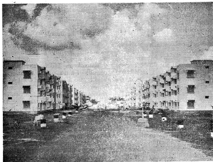
The Vyasarpadi Tenements built by Slum Clearance Board.
