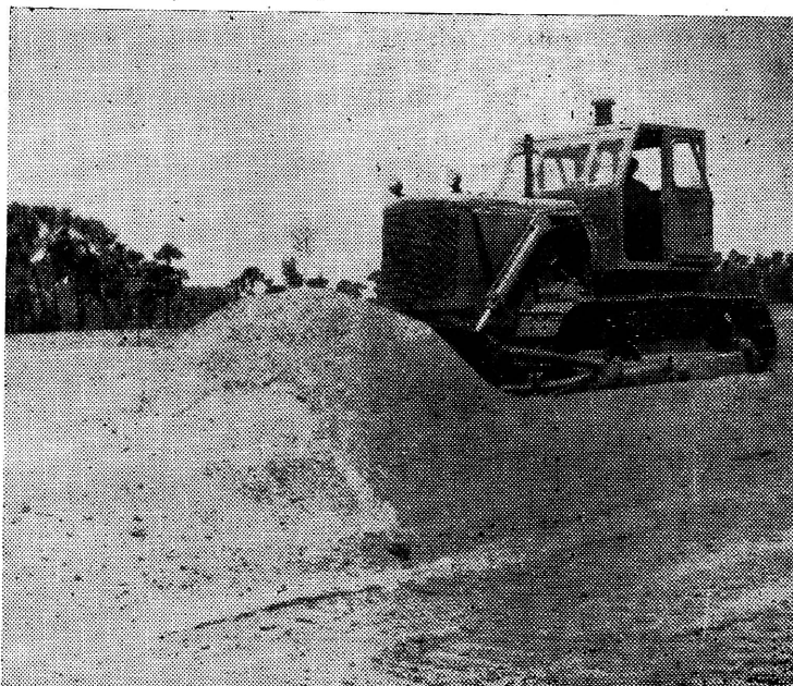
A bulldozer at work.
