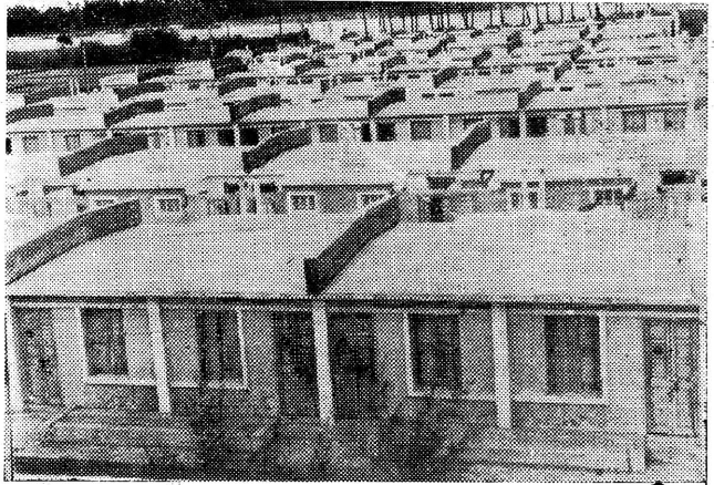
117 tenements for slum-dwellers constructed at a cost of Rs. 3 lakhs at Gundusalai road, Cuddalore.
