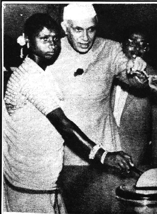
A woman worker dedicating Panchet Hill Dam across Damodar River, 6 December, 1959.
