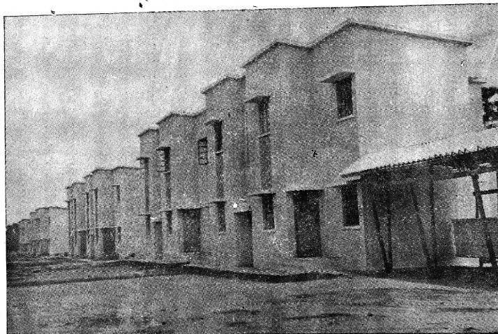
A batch of houses coming up at Avadi for Ordnance Workers.
