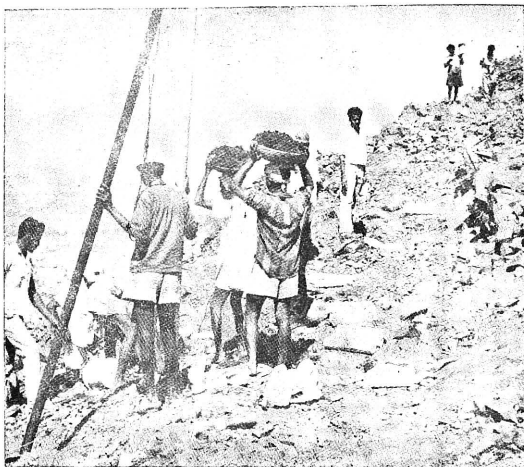
A pilot mine has been cut open in the Southern flank of the Kanjamalai hills to determine the behaviour of the mineral while blasting, the most suitable method of winning the iron ore and the equipment required for the purpose. The Neyveli Lignite Corporation Limited has been entrusted with the work of executing the pilot mine. Photo on top shows dynamite being put into the mine. Bottom photo shows the mine after the blast.
