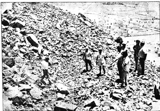
A pilot mine has been cut open in the Southern flank of the Kanjamalai hills to determine the behaviour of the mineral while blasting, the most suitable method of winning the iron ore and the equipment required for the purpose. The Neyveli Lignite Corporation Limited has been entrusted with the work of executing the pilot mine. Photo on top shows dynamite being put into the mine. Bottom photo shows the mine after the blast.
