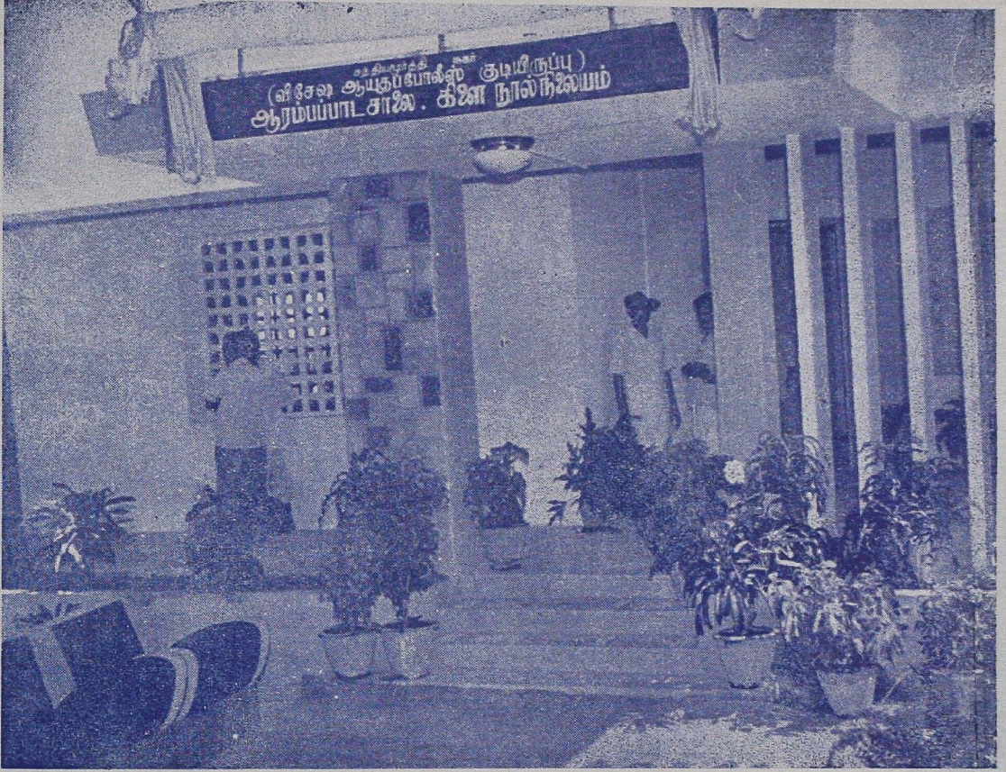
Entrance to the School Satyamurthi Nagar, Avadi.
