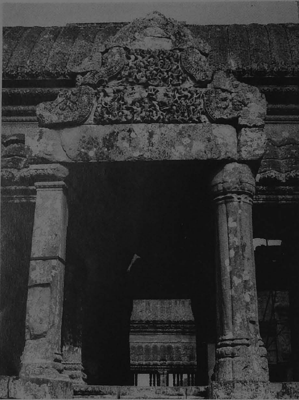
6. Gateway in second enclosure before treatment.
