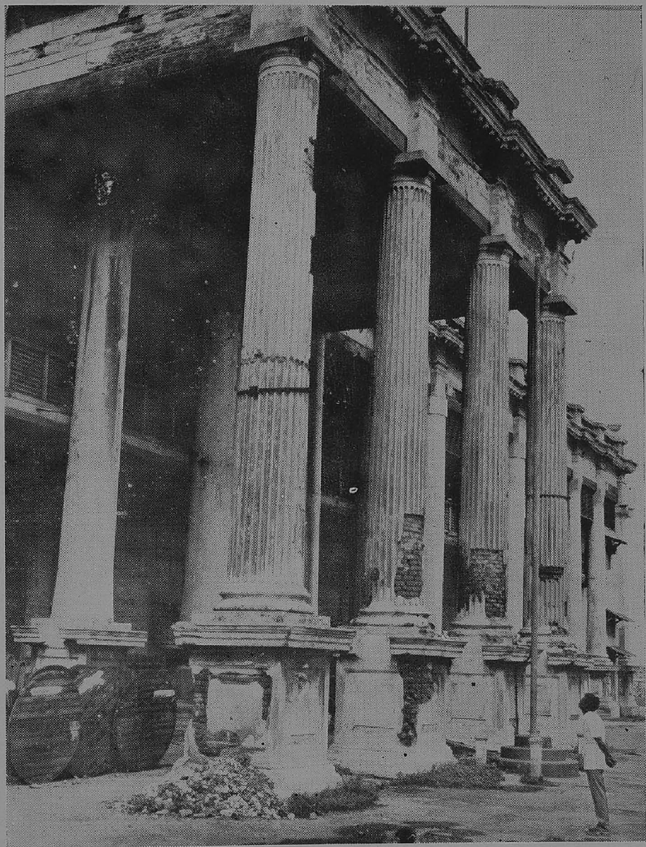
C : OLD RAILWAY HEADQUARTERS OFFICE. RAYAPURAM, MADRAS.
