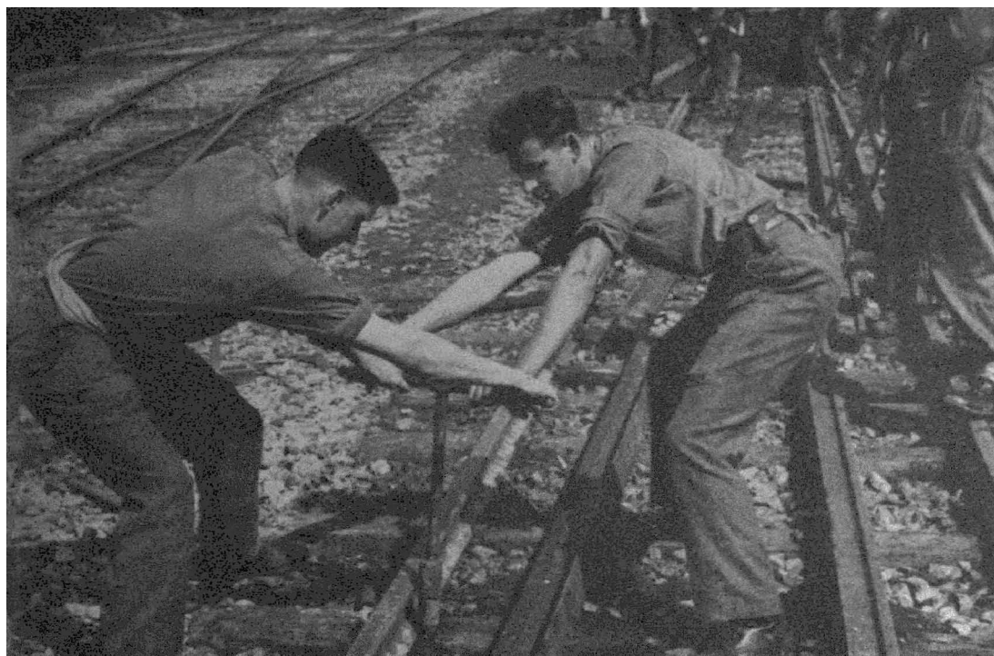
Royal Engineers laying new track in Tunisia
