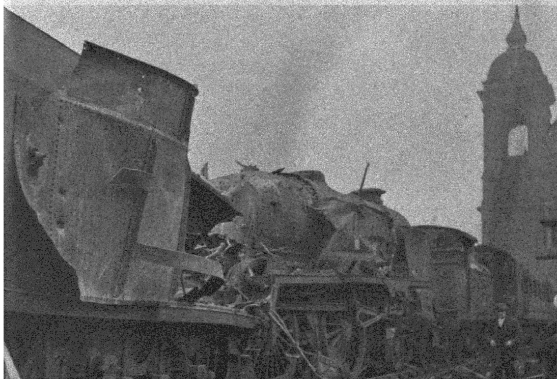
This 'Schools'-class locomotive took the full blast of a bomb and saved Cannon Street River Bridge from heavy damage
