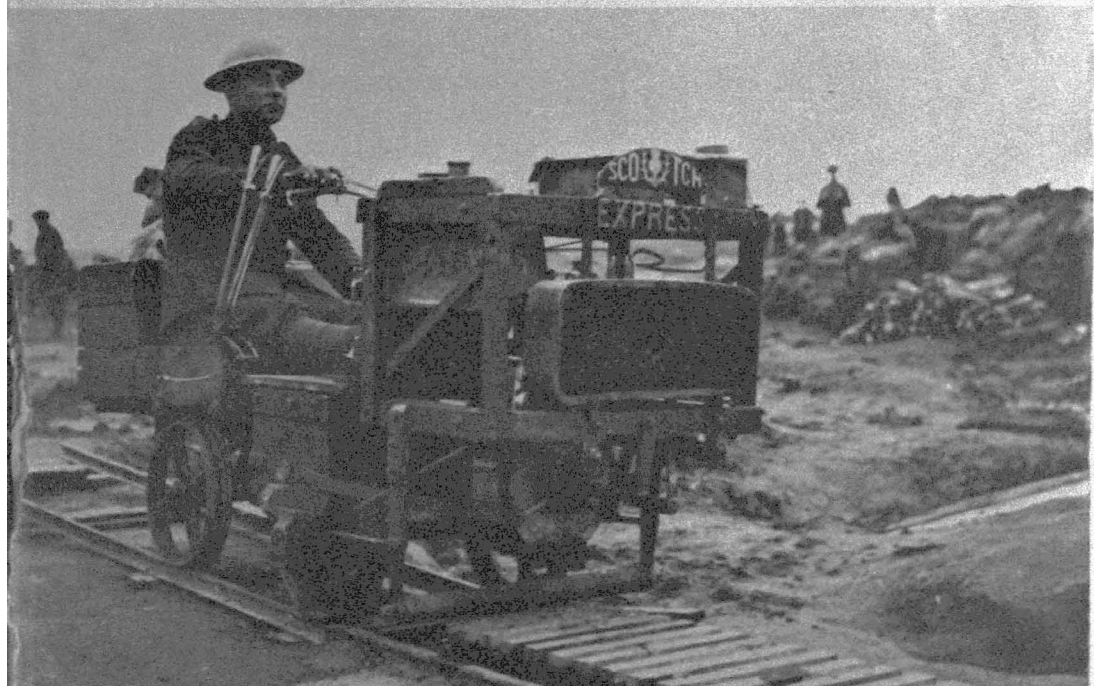
A First World War light railway 'engine' made from parts of a discarded motor car
