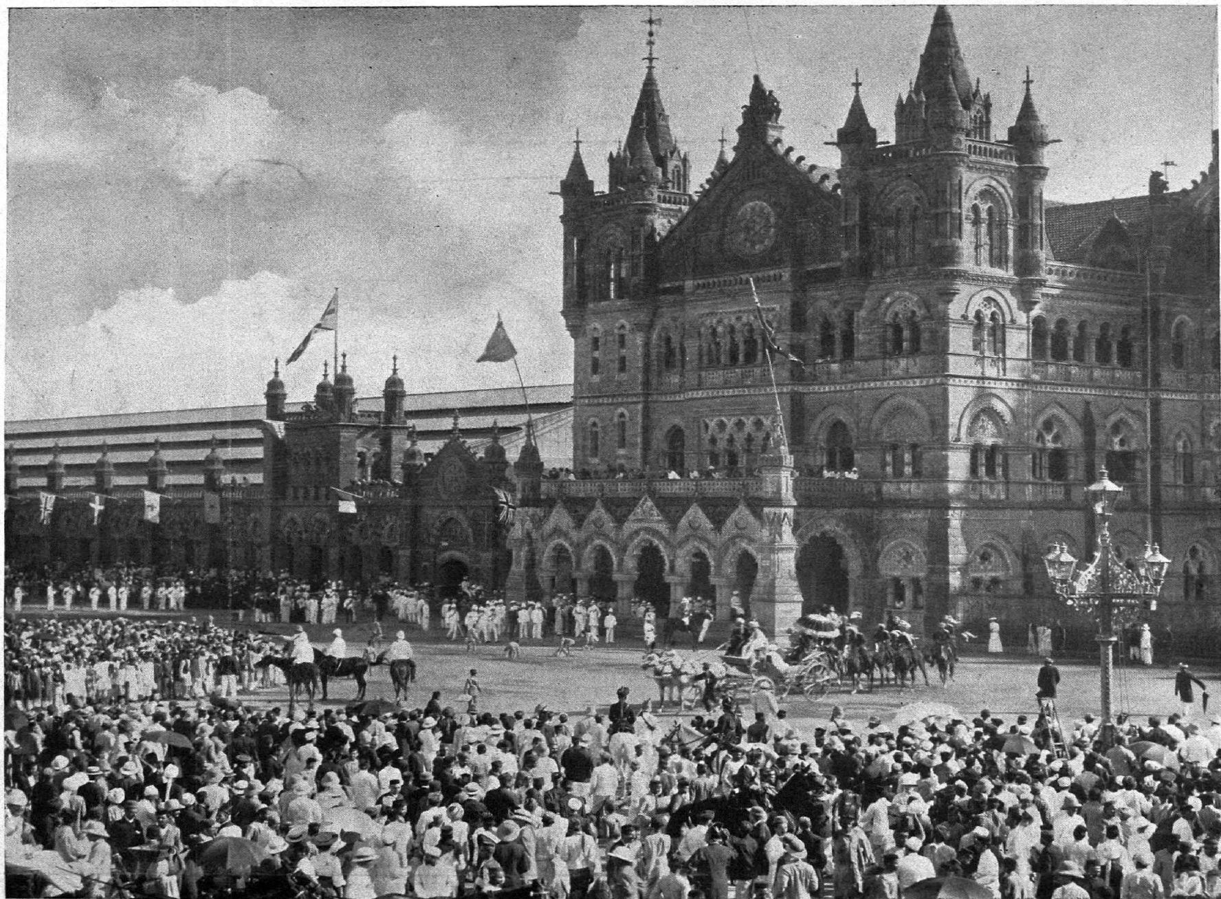
The G. I. P. Railway Station, Bombay.
