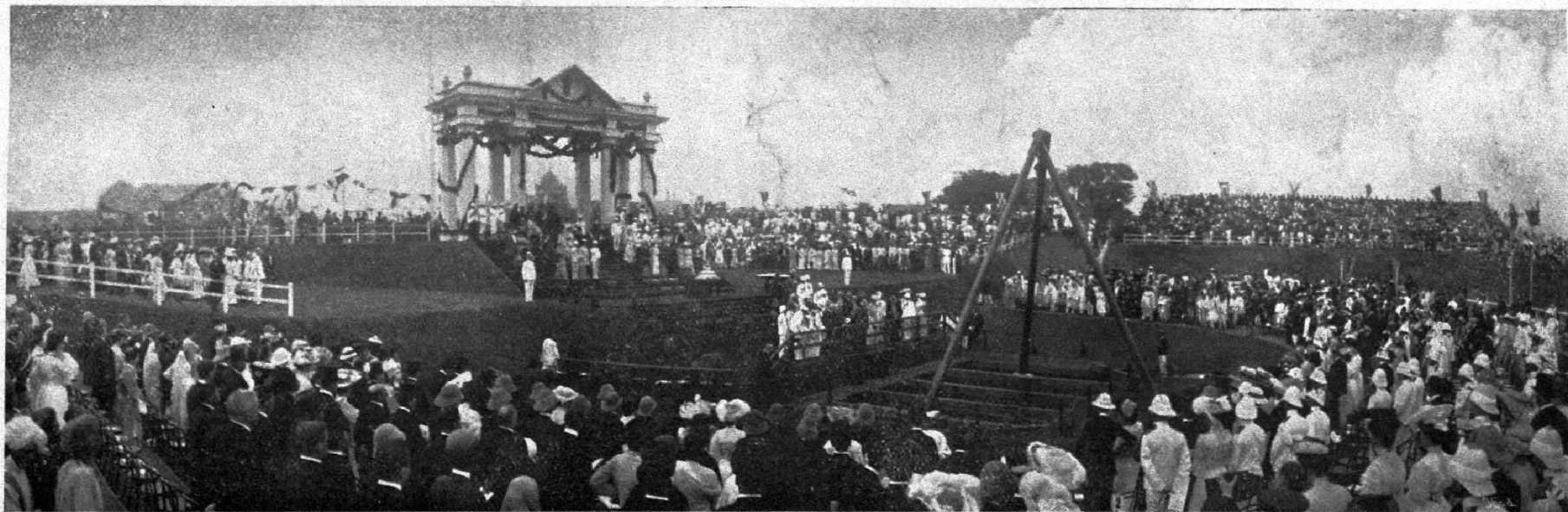
Laying the Foundation Stone of the Alexandra Dock, Bombay.
