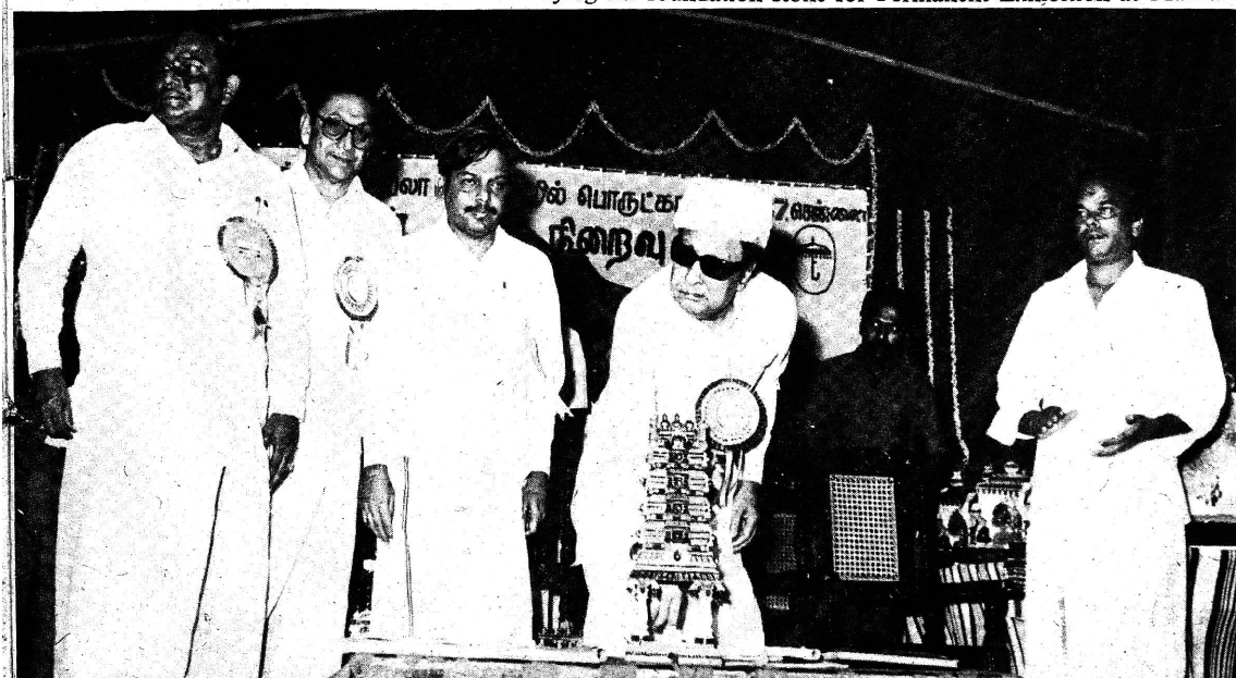
Laying the foundation stone for Permanent Exhibition at Madras
