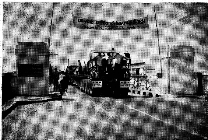
Photo shows the Load Test on Coleroon Bridge at Trichy. various aspects of Highways Engineering throughout the country. different soil, rainfall and water conditions?
