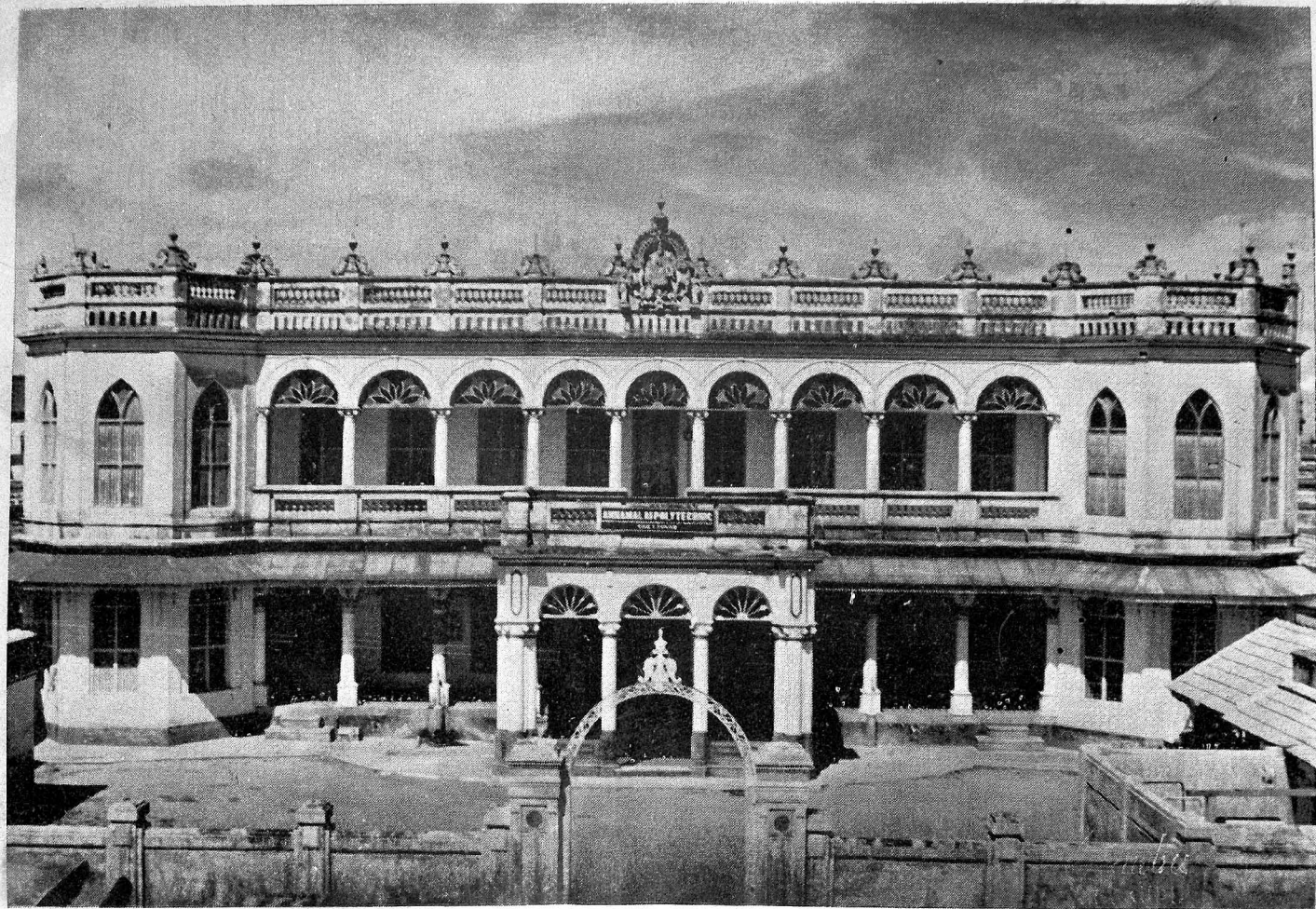
THE ANNAMALAI POLYTECHNIC, CHETTINAD TEMPORARY BUILDINGS
