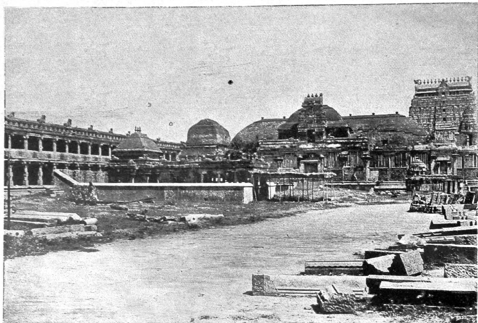
A view of west outer prakara with Sundareshwara Temple and 100-pillared mantapa.
