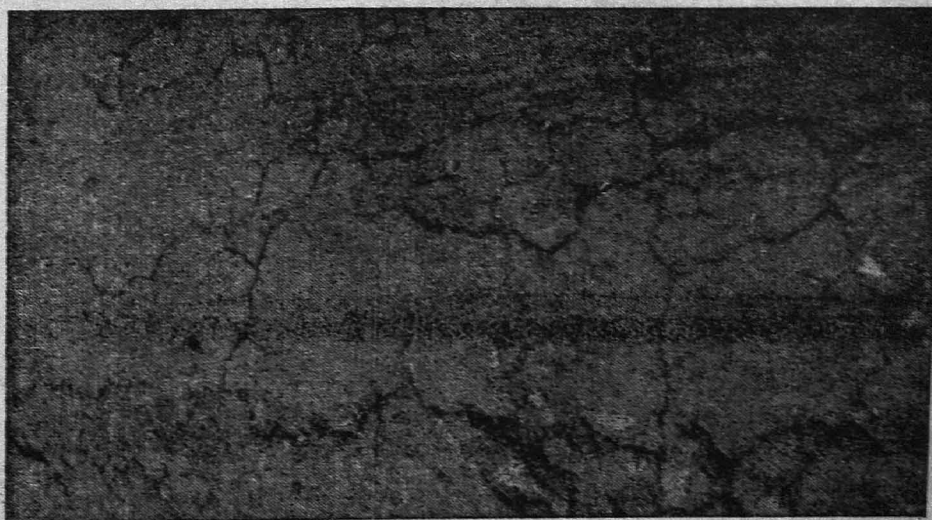
Fig 2.5.2. A close view of the distressed bituminous pavement in Mile 4/4 of Kumbakonam Kodavasal Road.
