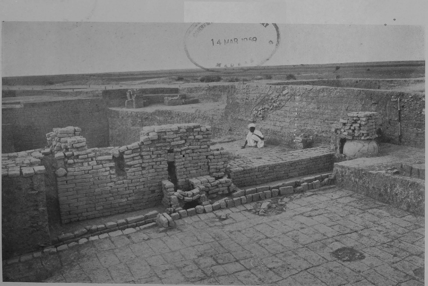
Fig. 5. Houses with drains and soakage jars, Lothal.
