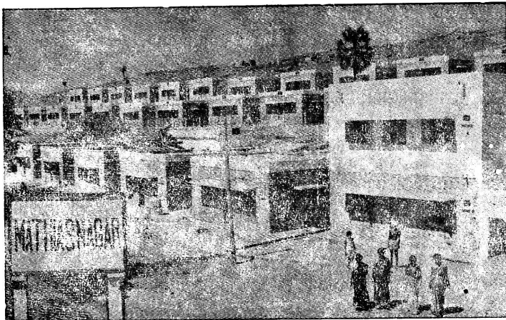
The overall view of Mathias Nagar a housing colony built for the Poor at St. Thomas mount.
